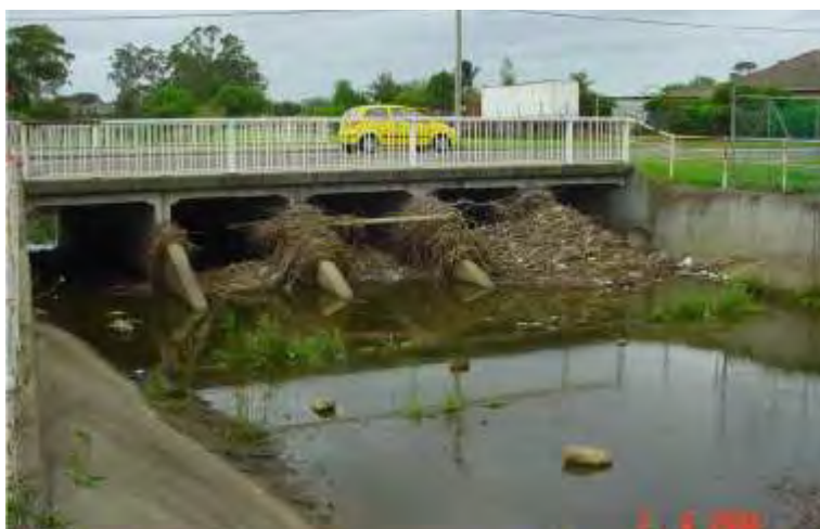
c. Blockage at Green Valley Creek at Cabramatta Road West culverts
