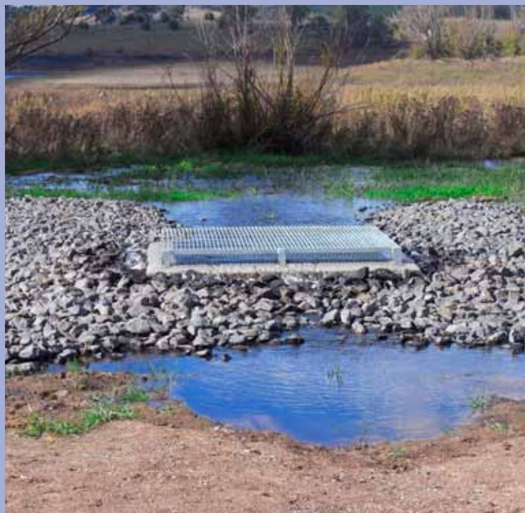
Harvested stormwater entering Suma Park Dam, Orange.
