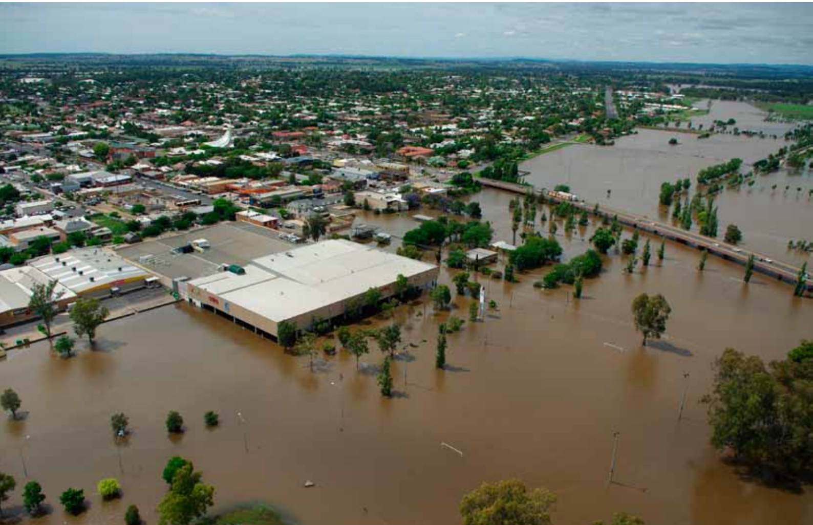
ABOVE Flooding in Dubbo CBD.
