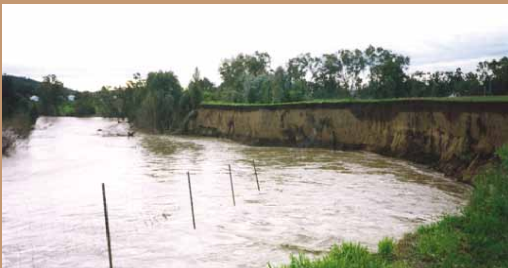
Riverbank erosion on the Bell River, Wellington.
